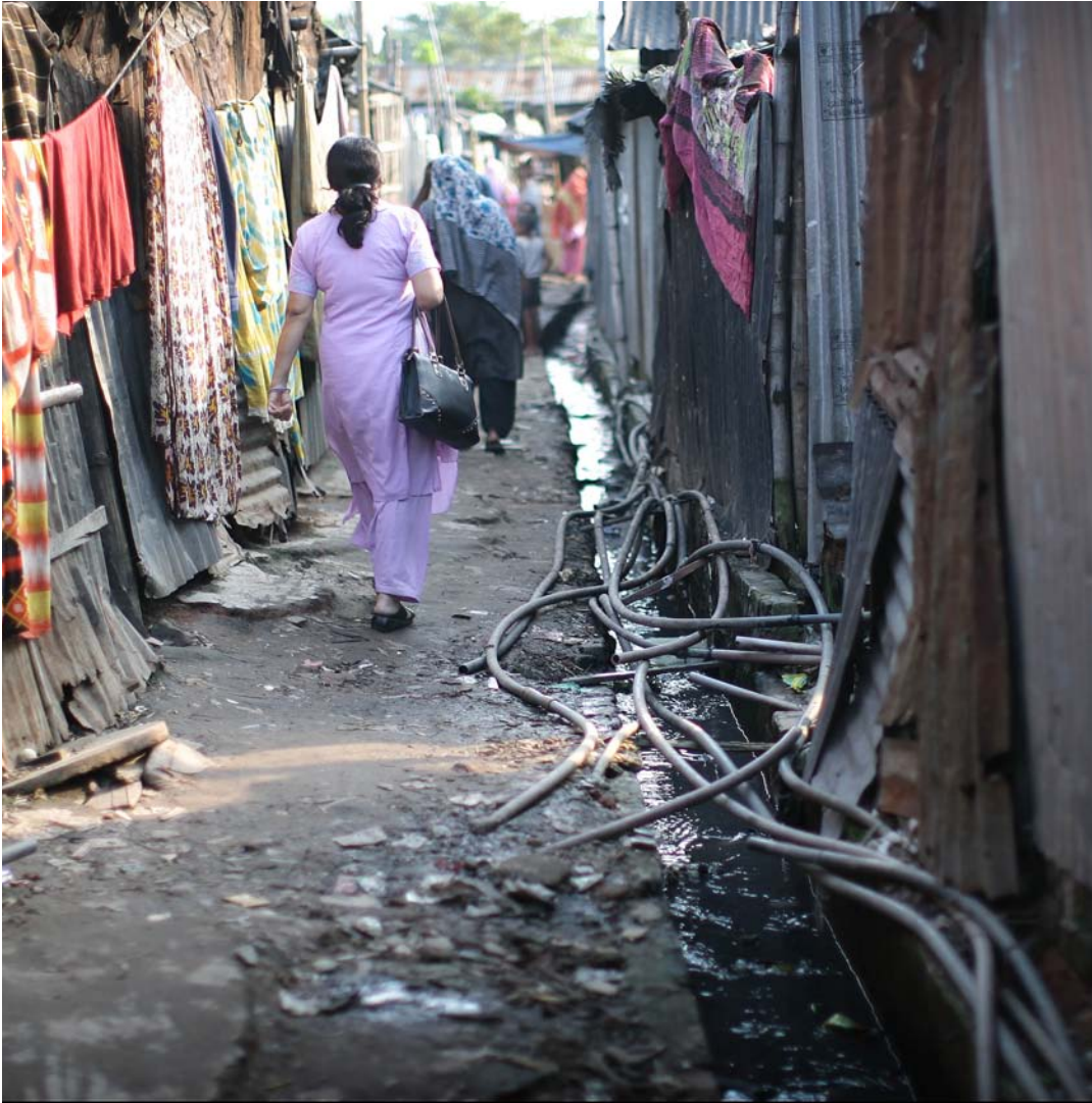
A tangle of pipes supplies water to unofficial water points in the Korail slum in Dhaka, Bangladesh.
