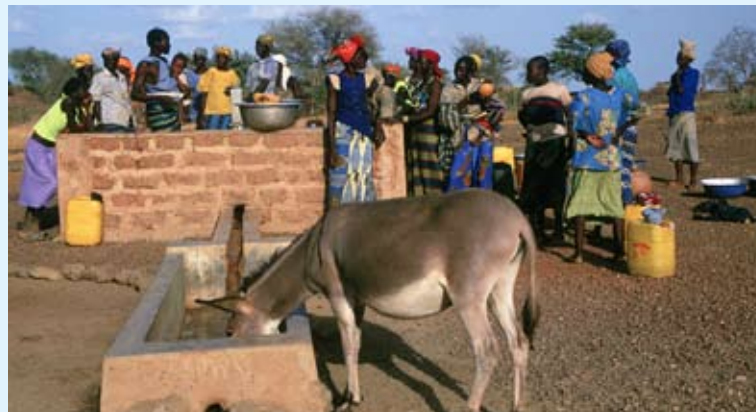
← ↑ The villagers of Yaké used the skill and knowledge of local well-diggers to construct a hand-dug well. They lined it with concrete to prevent pollution and protect it from collapsing in the wet season. Now everyone, the young, the elderly and even the community's animals, benefit.
