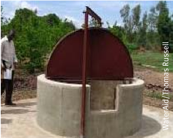
Picture 2: New well design for people who are blind, used by WaterAid in Mali
