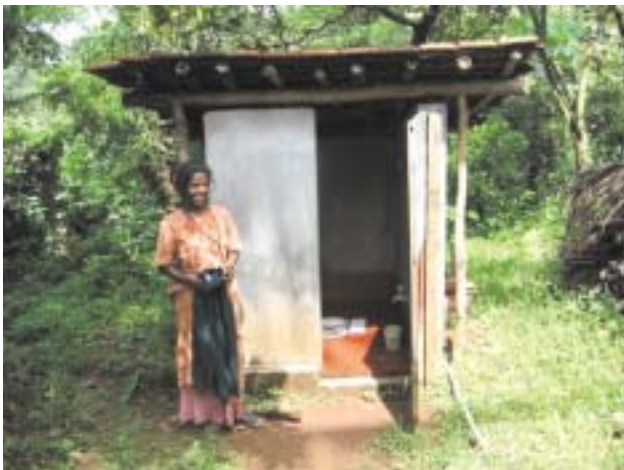
Upgraded toilet in Shimoga
