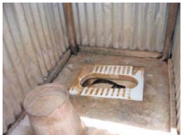
Toilet in a tribal village of Sarguja
