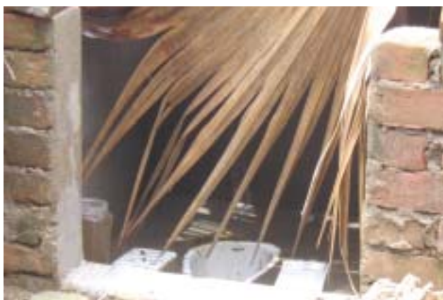
Latrine in Dalit household in Nalanda
