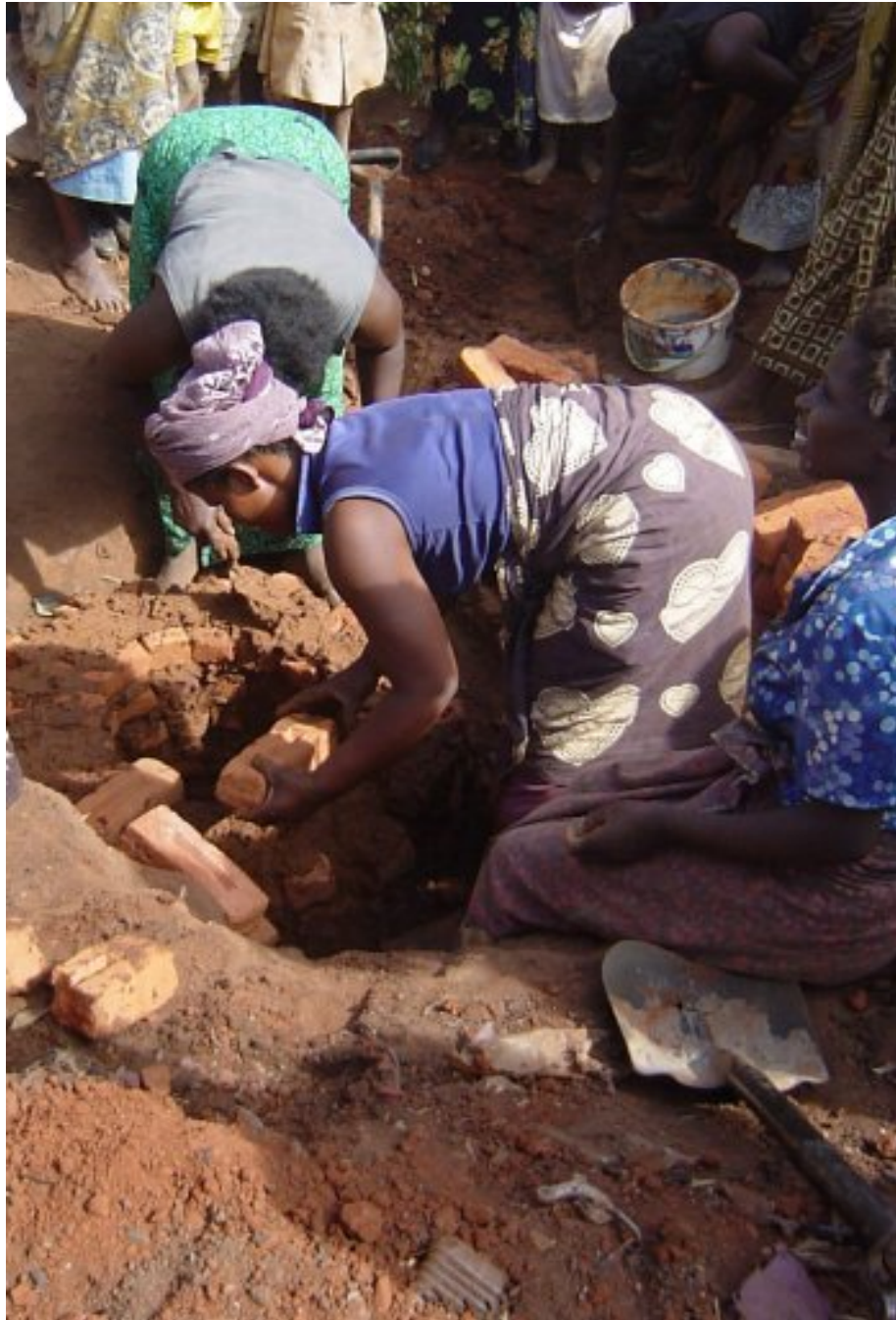
Women from low income areas lining latrine pits in Lilongwe Urban
