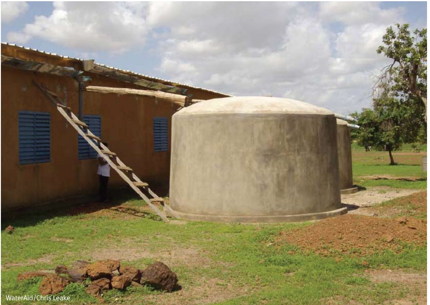
A rainwater harvesting tank at a school in Guirhora Kello, Burkina Faso.
