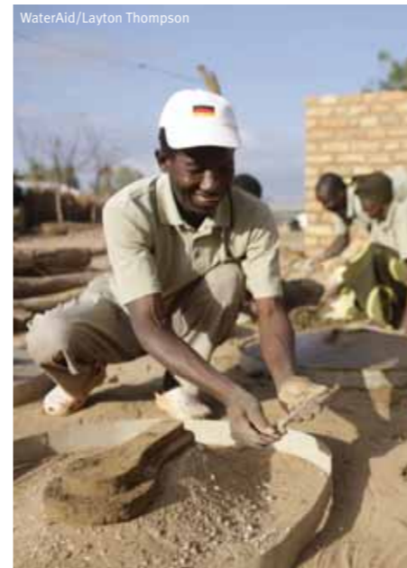
Kenedy Gondwe, a sanitation promoter in Malawi, making a latrine slab.
