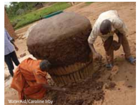
Building a rainwater harvesting jar in Uganda.
