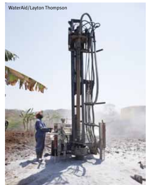
Drilling a borehole in Chiutika village, Malawi.
