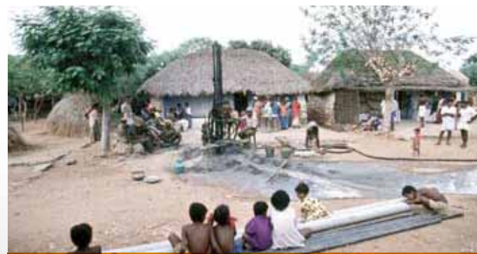
Drilling a well for water, India. Photo: WaterAid UK
