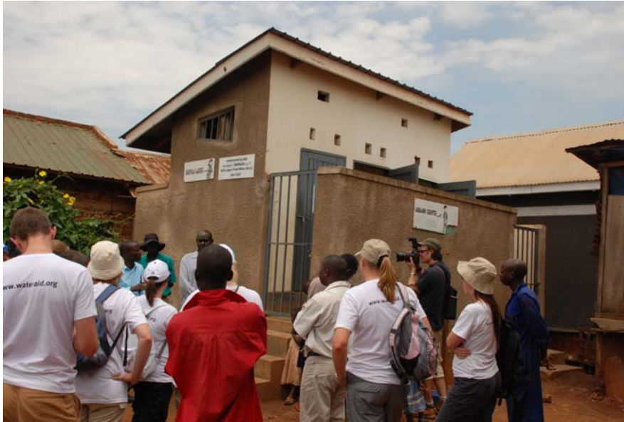
An improved toilet facility constructed with support from WAU
