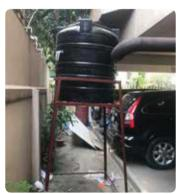
Water Tank (Capacity-500Ltr.) with support stand build with MS angle plumbing fittings Reservoir Brand: Gazi, RFL or any renowned brand
