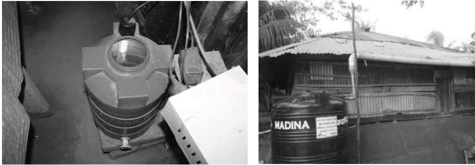
Figure 20: Application of solar-powered UV disinfection of harvested rainwater in a rural RWH unit in Bangladesh supported by CAFOD and DFID and implemented by ITN-BUET
