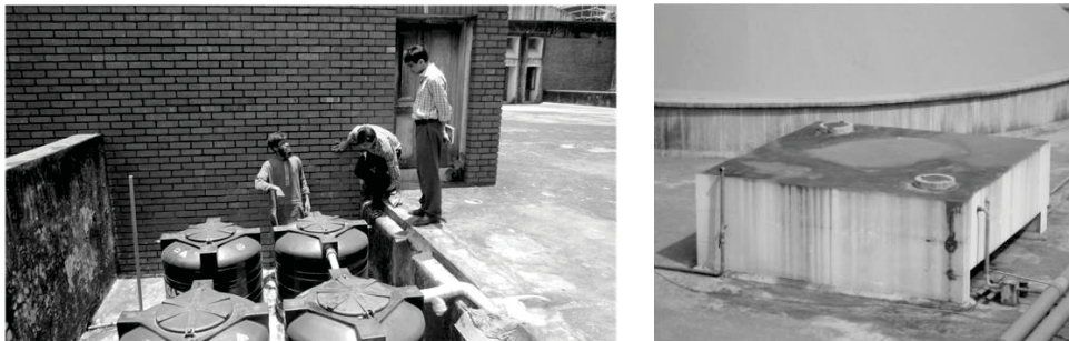
Figure 9: Rooftop rainwater storage tank arrangements at BUET cafeteria (left) and Independent University Bangladesh (IUB) (right)
