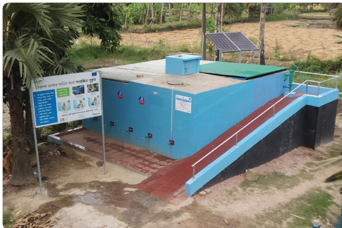
Image/ A solar-powered PSF plant in Shyamnagar, Satkhira which tops up safe water reservoir automatically.
