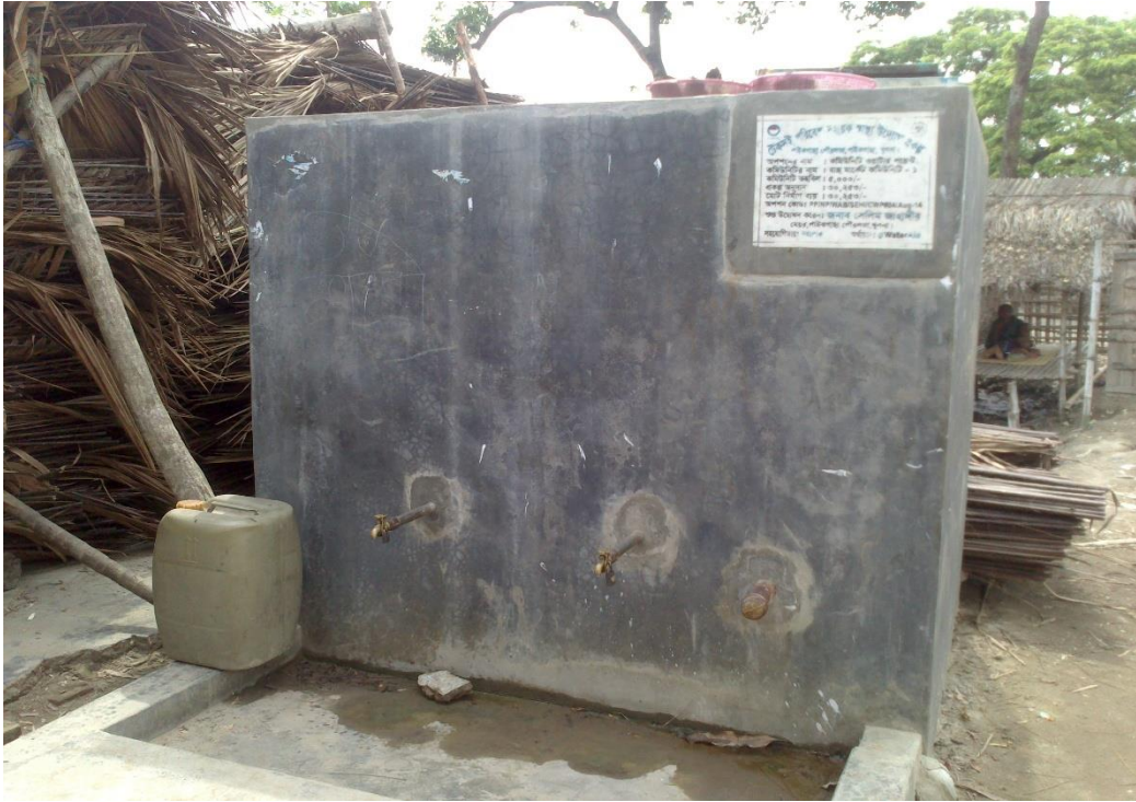
Picture 5: Community based Water Point at Paikgacha
