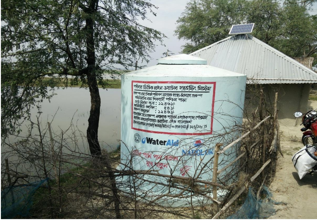
Picture 1: Household Rain Water Harvesting System at Paikgacha
