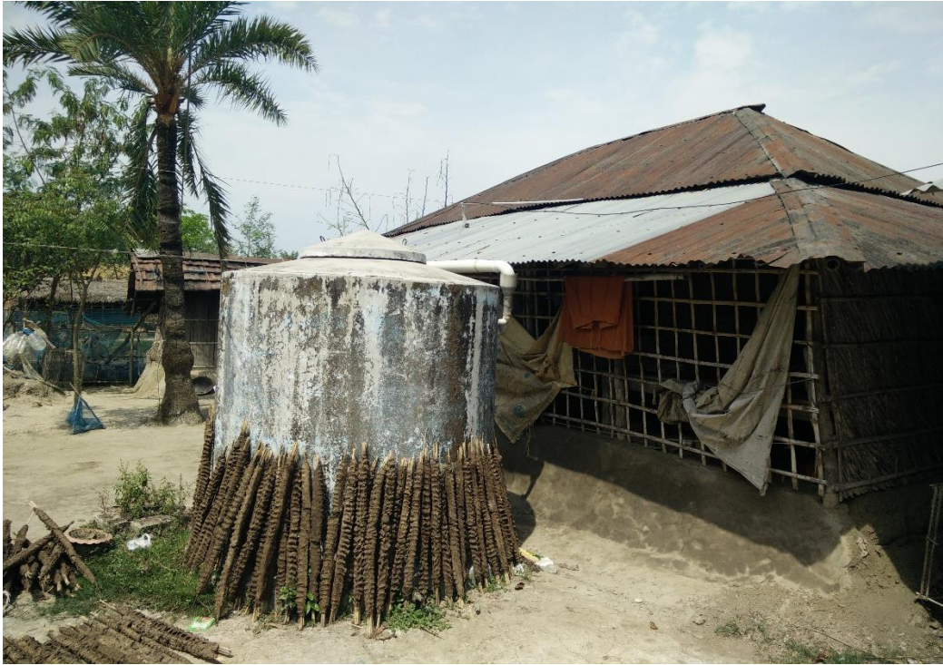
Picture 2: Household Rain Water Harvesting System at Paikgacha
