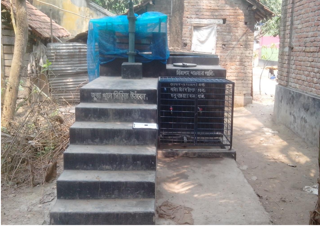
Picture 9: Community based AIRP unit at Kalaroa
