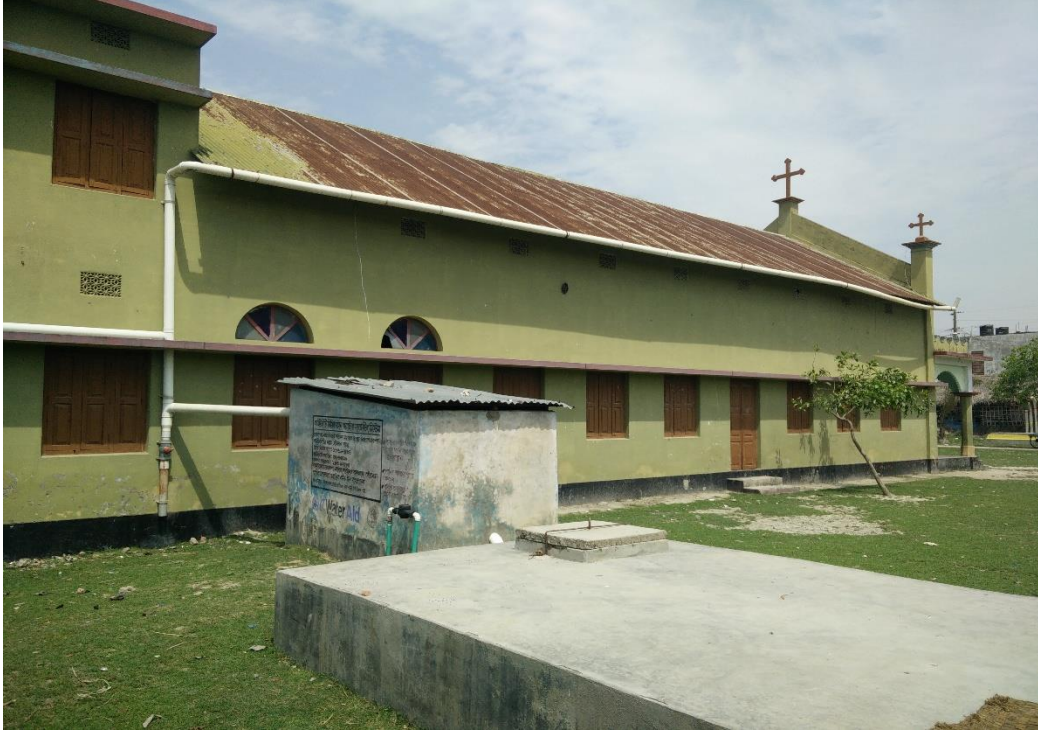
Picture 3: Community based Rain Water Harvesting System at Paikgacha
