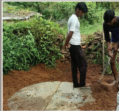
Small size covers also suffice due to corbeling
