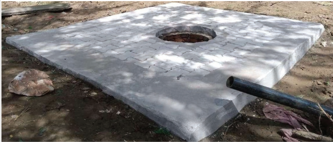
Completed unit with top layer of paver blocks
