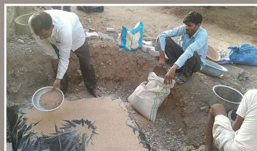
Covering pit with Polythene sheet
