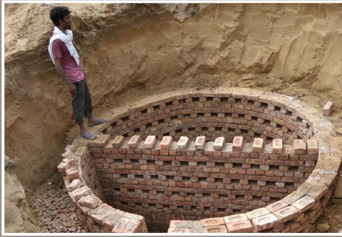
Leach pit under construction
