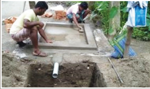
Making a washing platform near the soak pit
