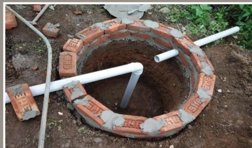
Brick-lined soak pit for rocky area with an overflow bypass
