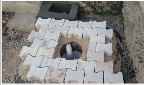
Paver blocks as final cover
