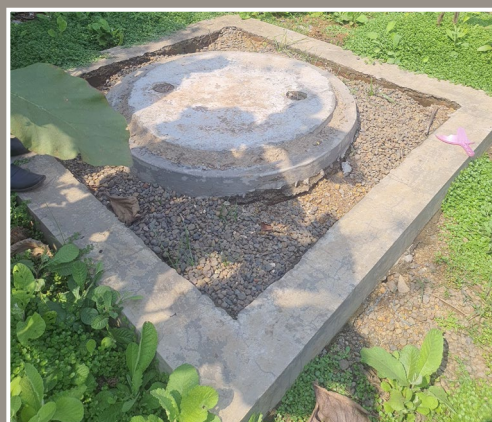
Additional brick-lined border to avoid flooding due to stormwater
