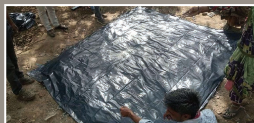
Laying polythene sheet over concrete
