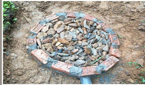
Soak Pit filled up to the upper layer with boulders.
