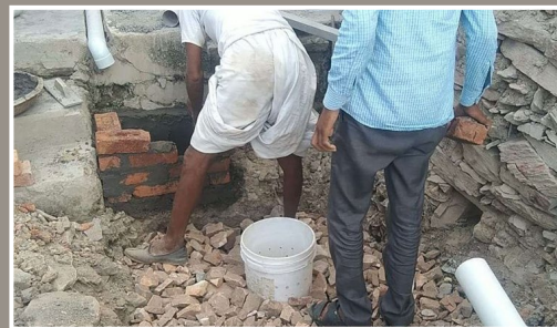
Placing plastic bucket and construction of chamber
