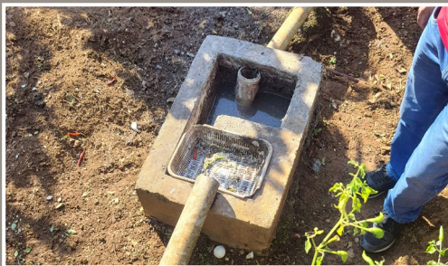
Plain plastic strainer required frequent cleaning
