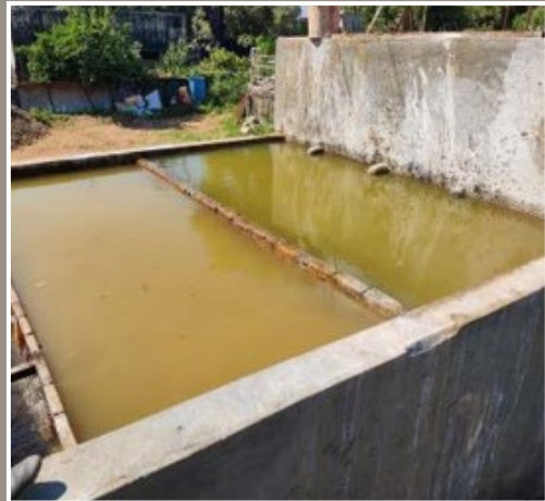
Settling tank no. 2 with activated charcoal
