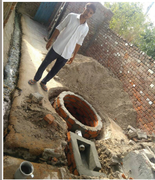
Leach Pit in Bhasada during construction in 2016
