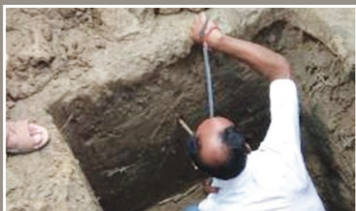
Excavation of the pit
