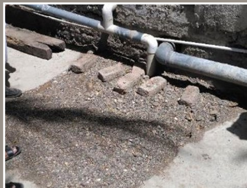
Filling with overburnt bricks (in place of boulders)
