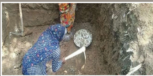
Excavation of Pit (7ft x 7t x7ft)
