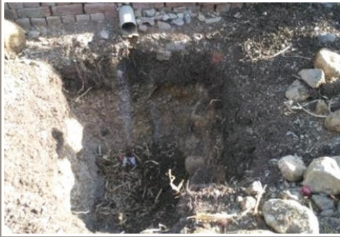
Excavation of the pit
