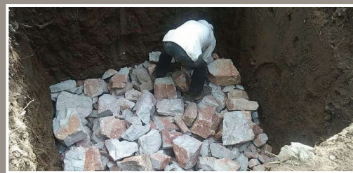
Filling with first layer of 200 mm stones up to 3 ft
