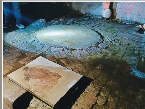
Leach pits in Bhasada in 2022- Functioning well
