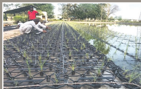
Typha plantation using floats
