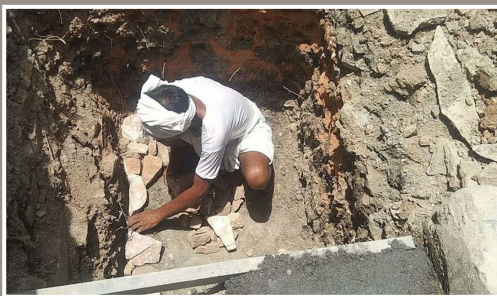
Excavation of the pit
