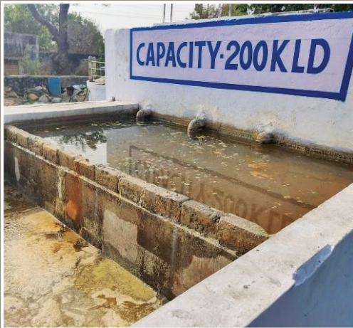
Settling Tank no. 1 with pebbles and large size charcoal
