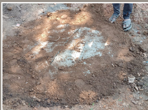
Leach pit covered with two semi-circular concrete slabs
