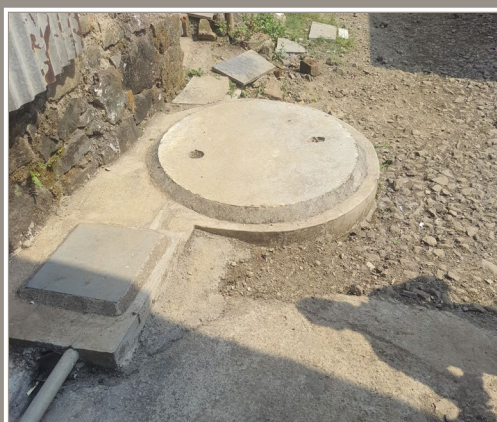
Completed community leach pit
