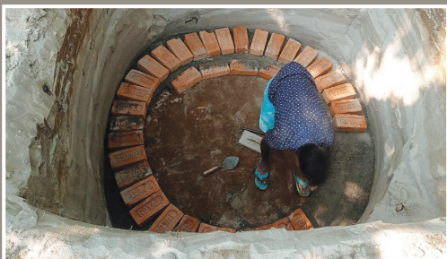
Community leach pit under construction
