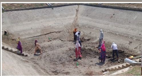
Operation & Maintenance of maturation pond
