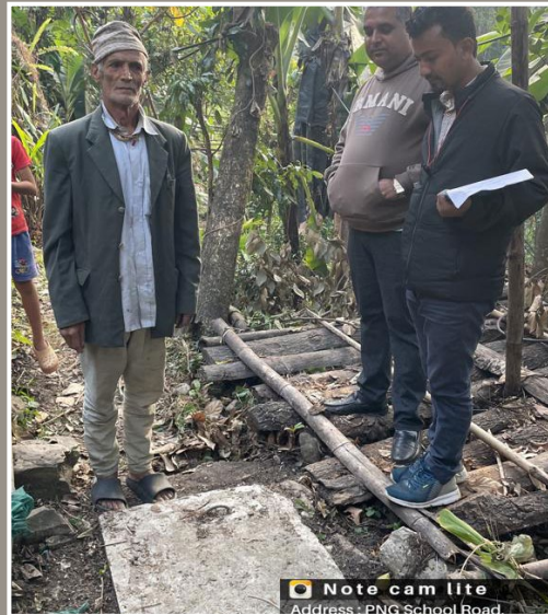
Soak pit covered with concrete slab
