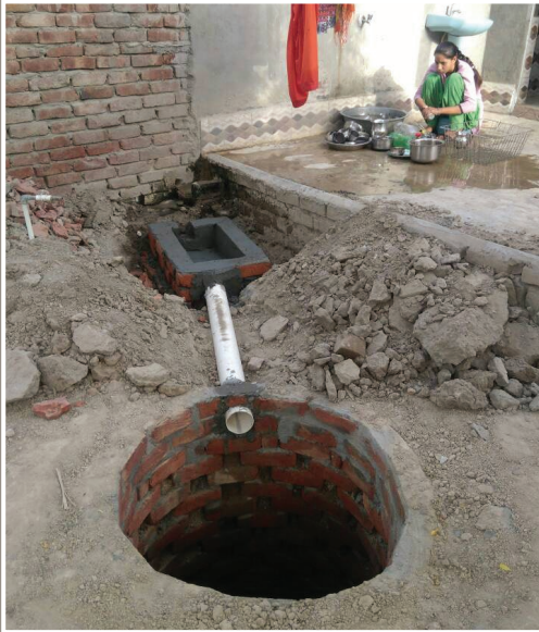
Leach Pit in Bhasada during construction in 2016
