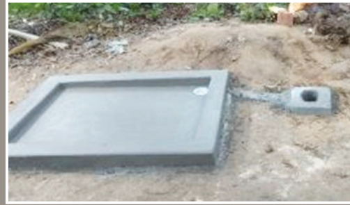
Completed soak pit along with washing platform
