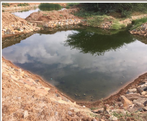
Settler tank with aerobic ventilation
