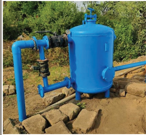
Granular filter-cum-doser for alum and lime
