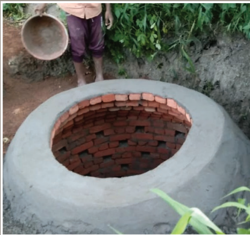
Completed community leach pit
