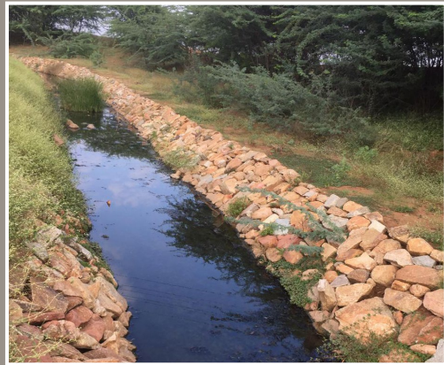
In-line convey channel to settler tank
