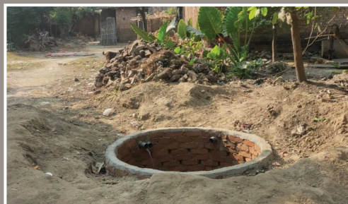
Community leach pit nearing completion
