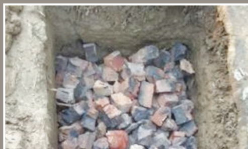
Filling with overburnt bricks (in place of boulders)
