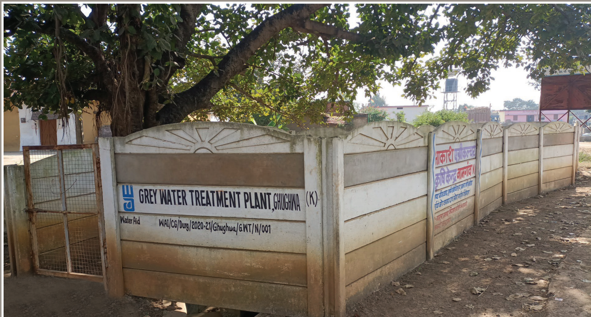
External View of DEWATS system
