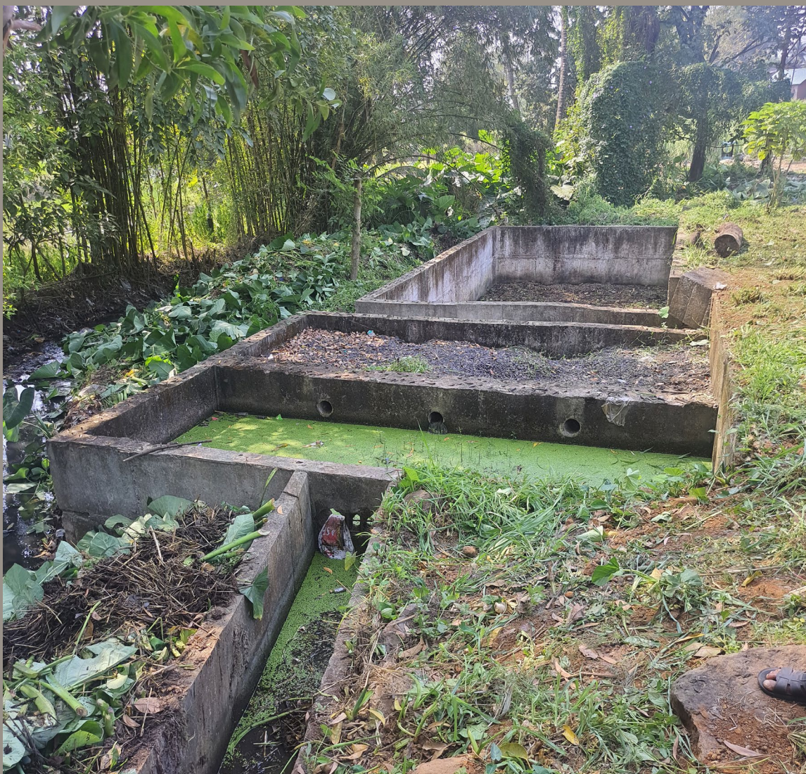
Bioremediation and Phytoremediation unit showing 1) Feeding channel 2) Collection-cum-settling tank 3) Bio Tower and 4) Bio-filter in a series
