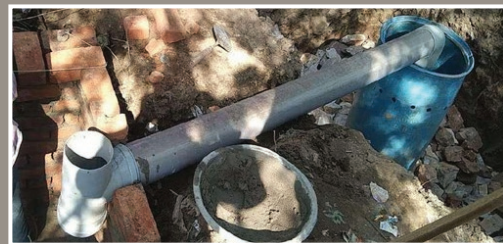
Construction of silt chamber and connecting pipe
