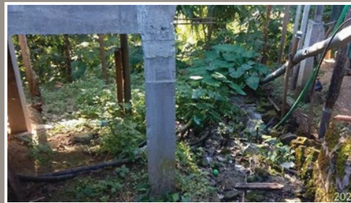
Each house has enough space below for gardening where the grey water is simply flown
