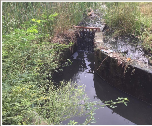
Screening and velocity baffle walls with pit
