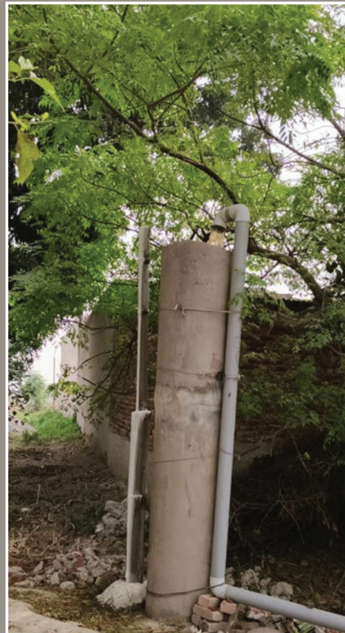
Raised tower for ease in irrigation by gravity
