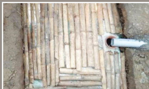
Making low-cost cover with bamboo pieces
