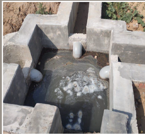
Branched silt chamber-cum-grease trap to arrest physical impurities and oil and grease
