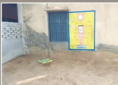
Community Magic pit with a connecting chamber (fully underground)
