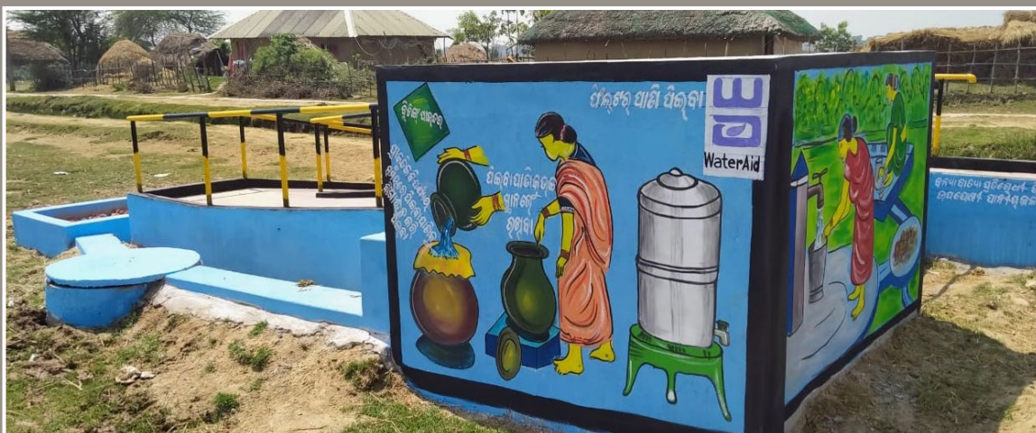
Raised washing platform, Soak Pit and a Reed Bed
