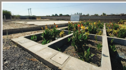
Planted Gravel Bed
