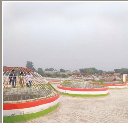
Digestion tank, Skimming Tank and Stabilization Tank all in series
