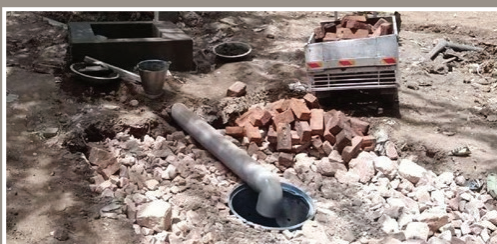
Second filling with stones around the drum
