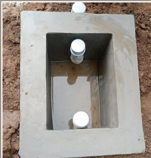
Well-constructed silt chamber
