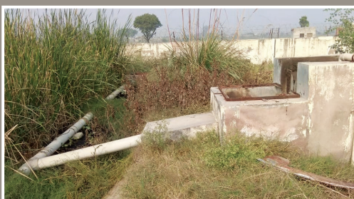
Distribution system with perforated PVC pipes
