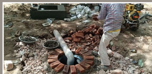
Construction of round neck around the drum
