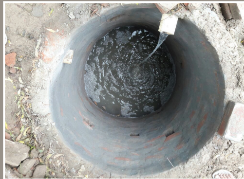
Leach Pit commissioned (cover removed for observation) 2016
