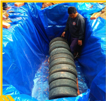
ARRANGING OLD TYRES TO FORM A TUNNEL
