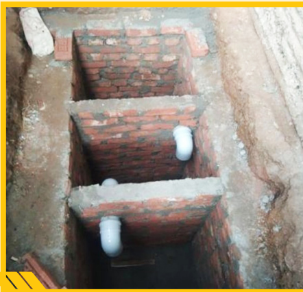
PARTITIONS FOR CHAMBERS AND PIPE FITTING
