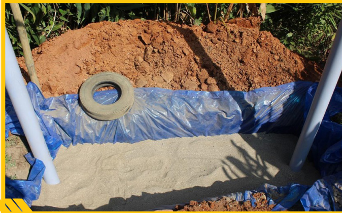
PUTTING SAND LAYER
