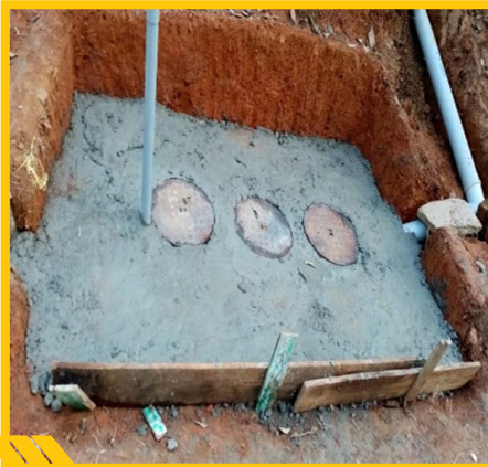
VENT PIPE FITTING
