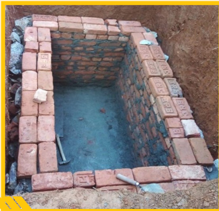
CONSTRUCTION OF TANK WALL
