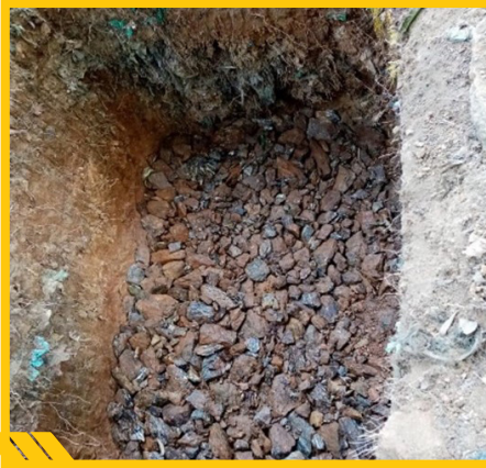
FILLING UP THE PIT WITH AGGREGATE FOR THE BASE
