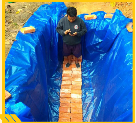
PUTTING BASE OF BRICKS
