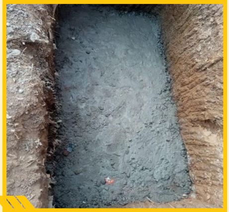
CREATING THE BASE WITH CEMENT CONCRETE
