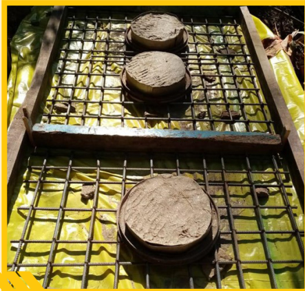
CONSTRUCTION OF TANK SLAB WITH INSPECTION HOLES
