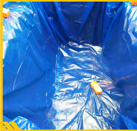
LINING WITH HDPE SHEET
