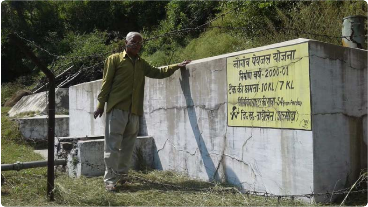
The Inar water supply project was based on a demand-driven participatory approach.
