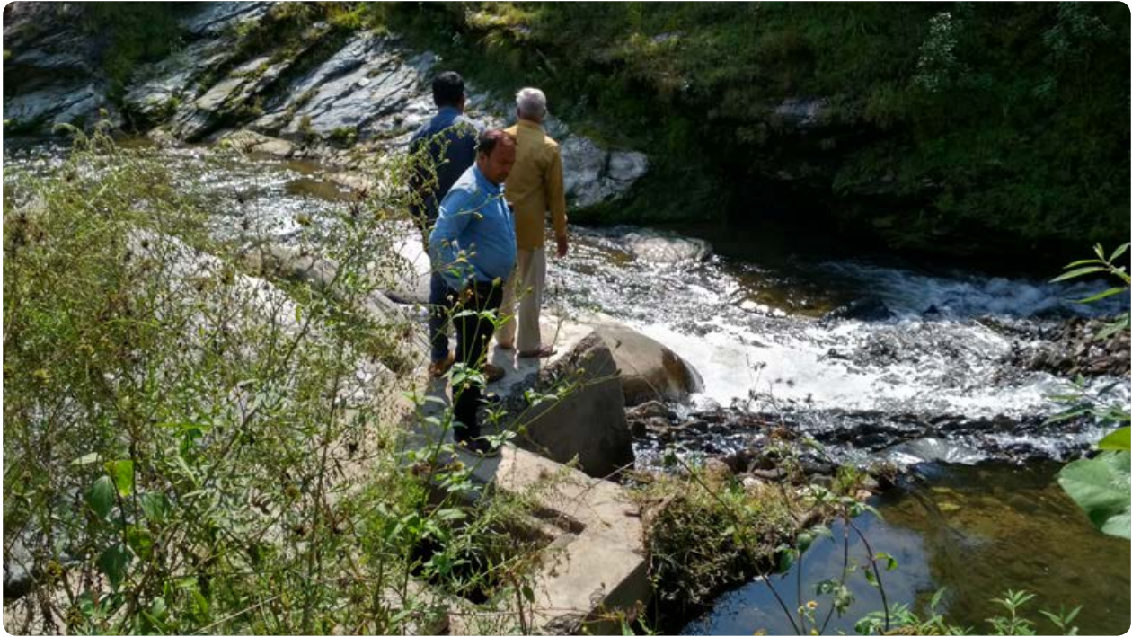
Inar water supply project's intake source. Periodic cleaning of the boulder-filled gallery and replacement of boulders is undertaken in order to provide sustainable water supply.
