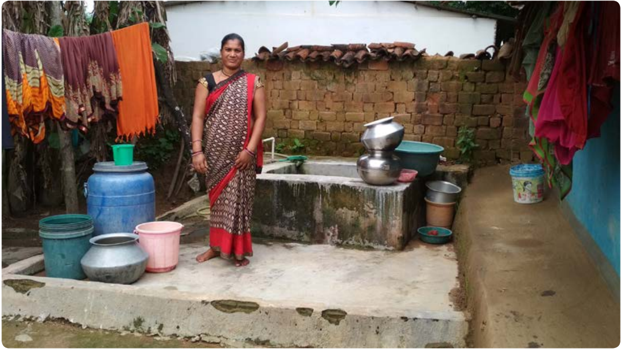
Water supply system at household level
