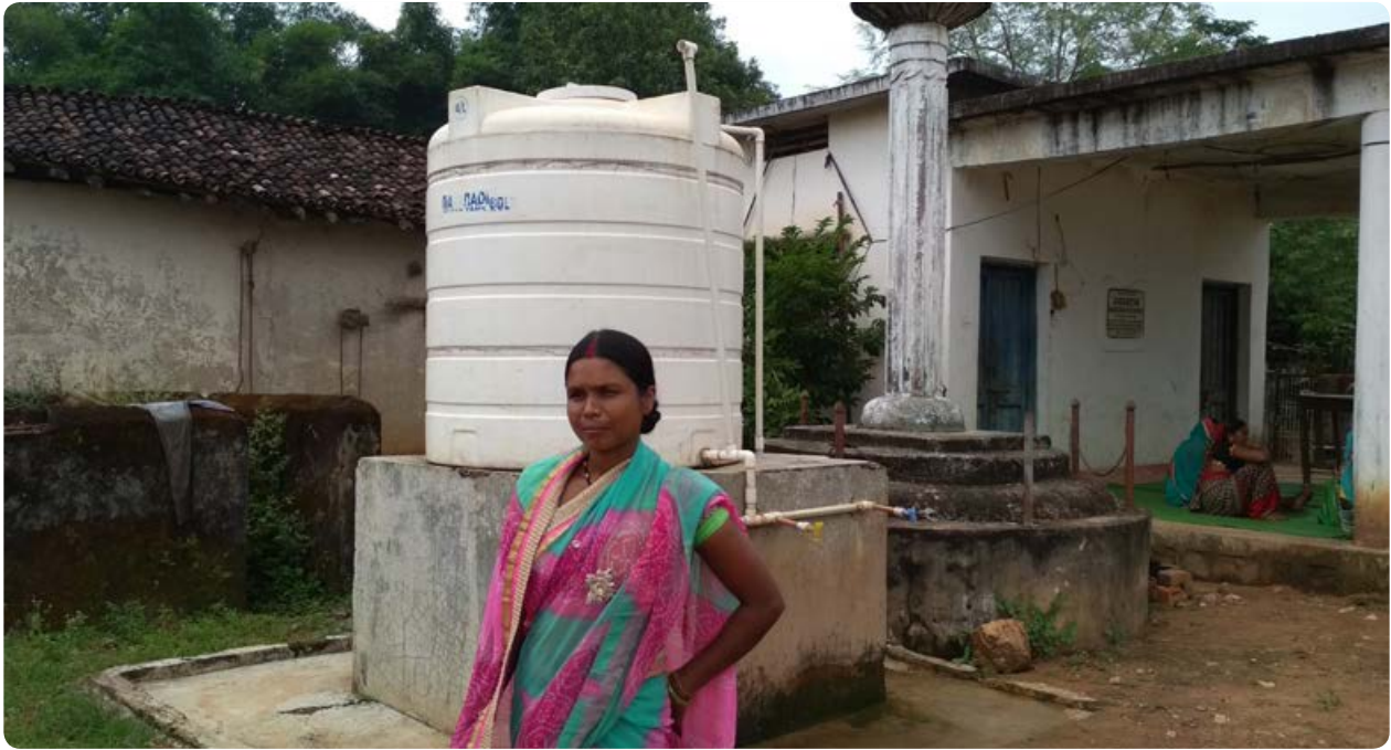
The piped water scheme at Sivani main village
