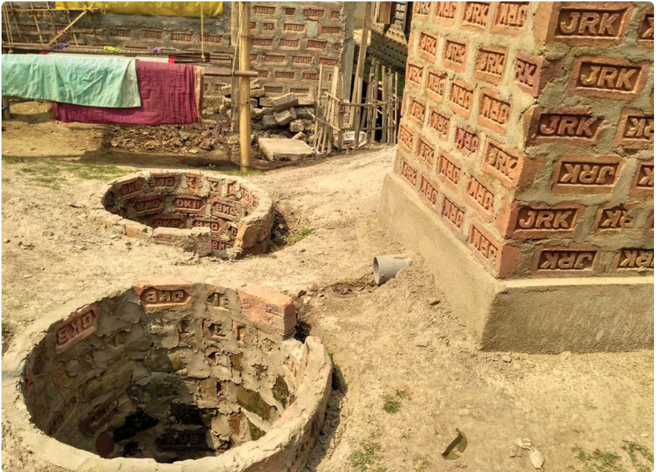
A faulty twin pit toilet structure.
