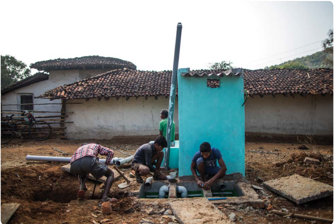
A bio-toilet under construction in rocky terrain of Hahaladdi village, Kanker, Chhattisgarh.
