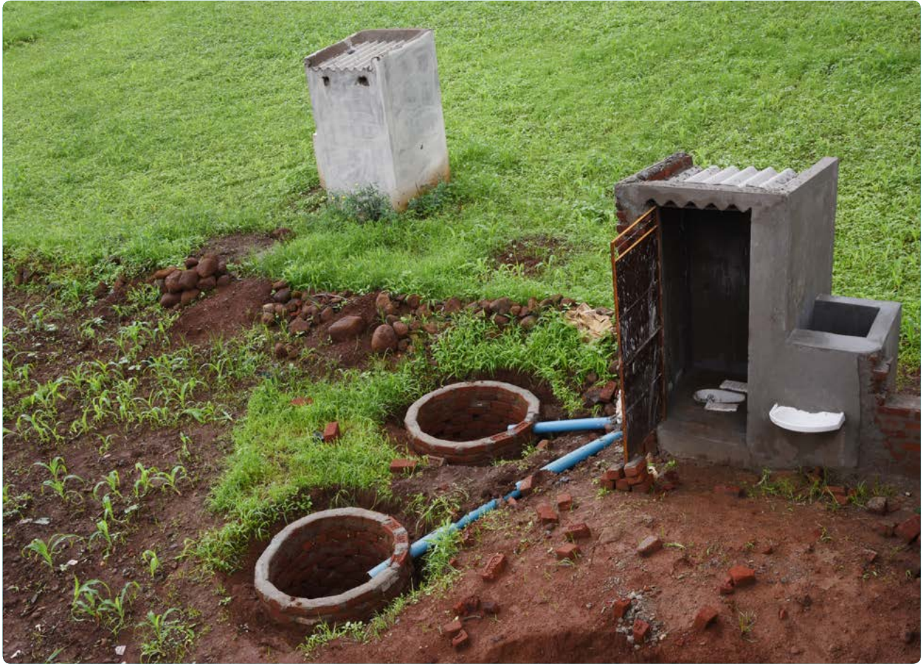
A twin leach pit toilet under construction in Padhariya Village, Dindori, Madhya Pradesh
