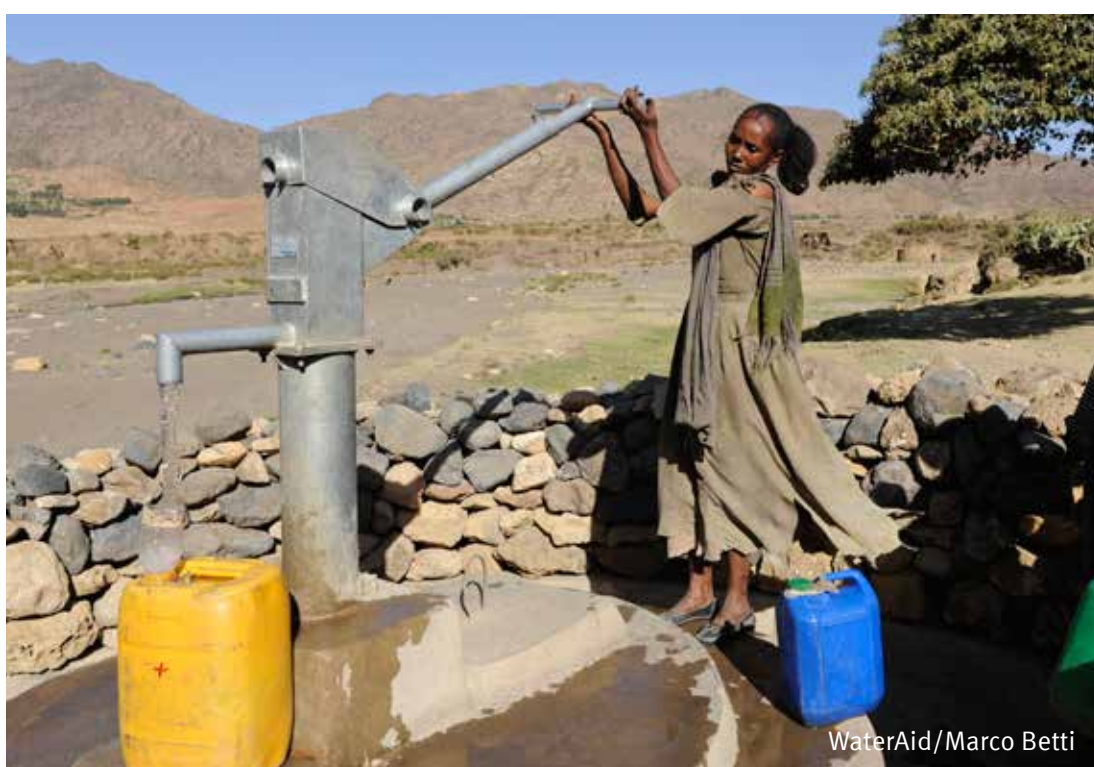
An example of a handpump operated hand-dug well with an apron and drain surrounding the well head in Adi-awna-waza village in the Hintalo-Wajarat region of Ethiopia
