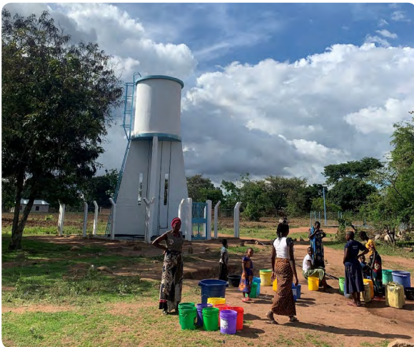
▲ Women carrying water outside the water tank in Nyamalimbe HCF, which also serves the community
