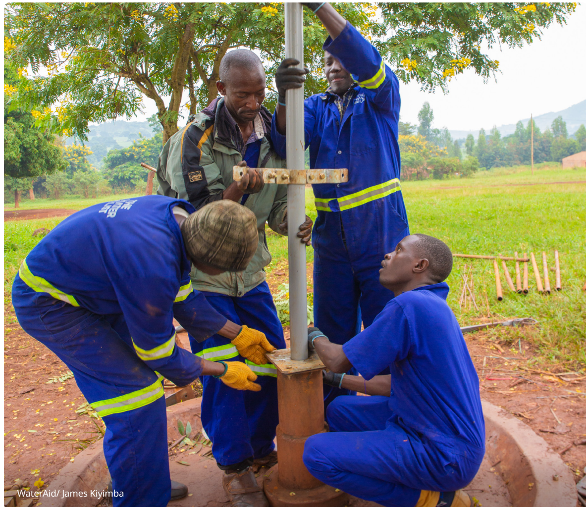
● Mechanics fit a PVC pipe to a handpump at Rukondwa Primary School in Masindi District, Uganda.
